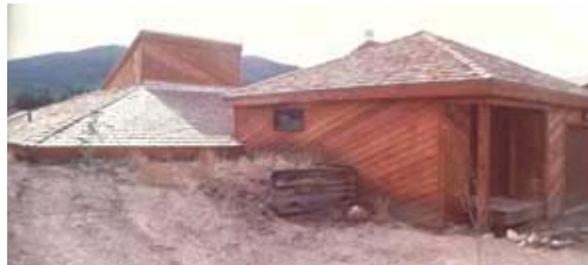
**While the Colosol structure's garage and air-lock entry way are located above ground, and the living area is set partially below ground and is partially earth-sheltered.**
