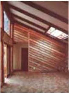
One of three Zomeworks Skylids helps to cast natural light into what would have been a dark living room corner. The strings which dangle from the Skylid offer a manual override of the device's solar-activated operation
